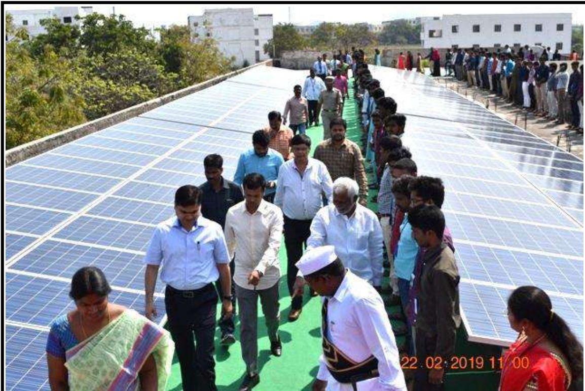
Solar Power Plant
